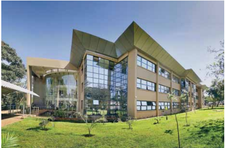
UN-HABITAT's new Nairobi home.
